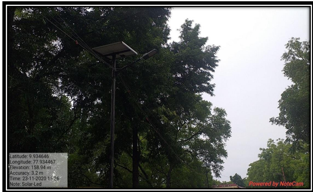
Sensor- based Solar LED Street Light near Car Parking (Capacity 25W)
