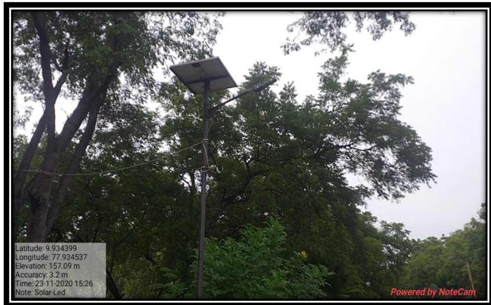
Sensor- based Solar LED Street Light near Car Parking (Capacity 25W)
